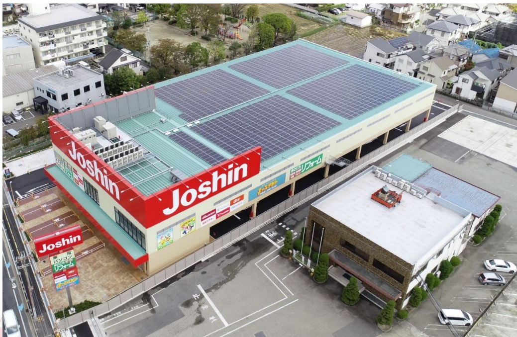
Appearance of Ibaraki Store (Opened in November 2019)
